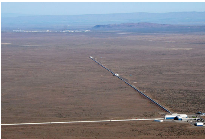
Fig. 16.3 Aerial photograph of the LIGO Hanford facility, showing the 4 km long arms of the interferometer. (Credit: Wikimedia Commons [3])
